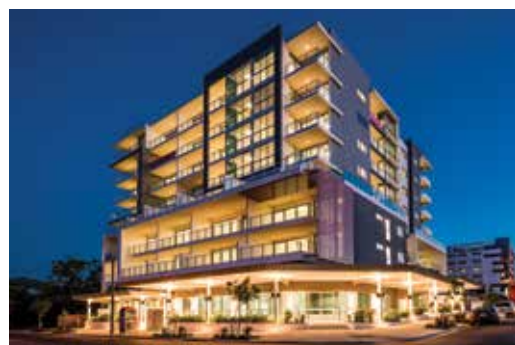
THE LINK NUNDAH, BRISBANE – COMPLETED 2016
