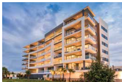
ETESIAN AT HARBOUR QUAYS HARBOUR QUAYS, GOLD COAST – COMPLETED 2013
